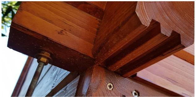
• If your garden house has a canopy with support post(s), it should be measured, cut to size and positioned on the post footing so that the pillar is 8cm higher than the terrace. This secures access to the post footing for later adjustments. The post footing is adjusted with the nut
