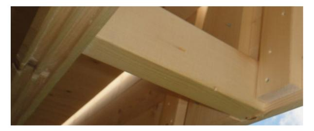
Parapets for larger cabins may consist of 2 or 3 pieces. Use parapet connecting strips to screw them together.
