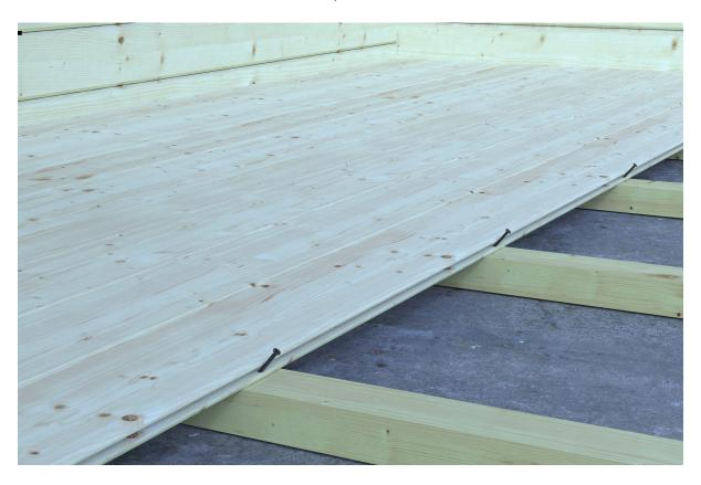
The few mm difference between the end of the floorboard and wall will not be seen after you install the skirting laths in the next stage. Some floorboards and the last floorboard must be cut into size. Avoid stepping on untreated floorboards with shoes to avoid footprints. Removal of footprints from untreated wood is very time consuming.
