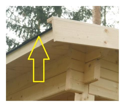
Afterwards, mount the gable boards and cover strips to the roof by using screws.
