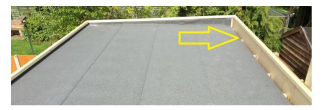
Some of our pelmets have vertical strips on the back side for strength. Before installing the front wall pelmet, you must cut sockets into roof boards for strips to go in. This will allow you to install the parapet tightly to the roof in the higher end of the cabin. Alternatively, you can reposition these connecting strips to outer side of the pelmets and install them without cutting the sockets.
