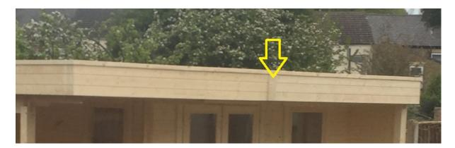
Pelmets must be screwed to rafter ends on the side walls and to the gable elements in the front and back side of the cabin. Front and back side pelmets must be additionally fixed to walls by using wooden parapet connecting supports. Use screws.
