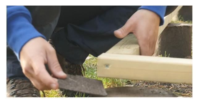
Alternatively, you may use a bitumen layer below the entire foundation frame. In that case, we recommend drilling 10mm wide ventilation holes into the frame from the sides with approximately 1 meter distance between the holes. This will create ventilation for eliminating moisture.
